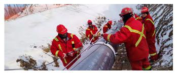
Fiber optic cables installation for the PLMS (pipeline leakage monitoring system) by Cameco
